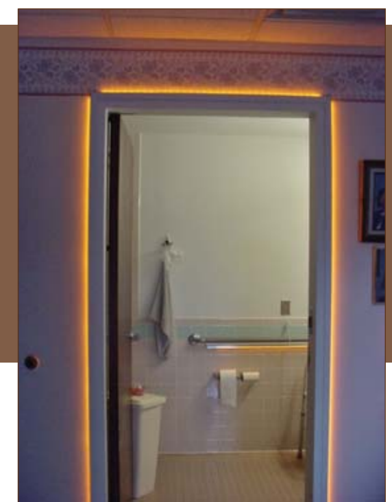
(Figure 9a) Delineation of transition zones. Horizontal and vertical lighting provides perceptual cues to help older adults orient themselves when awaking from sleep. These amber LEDs are photosensor and motion controlled. Amber was selected because it gives enough light to see and is closest in color to the familiar incandescent.
