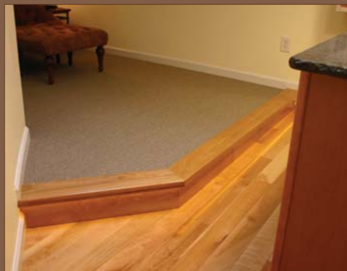
Figure 9b: Change in grade is marked by linear LEDs under step
