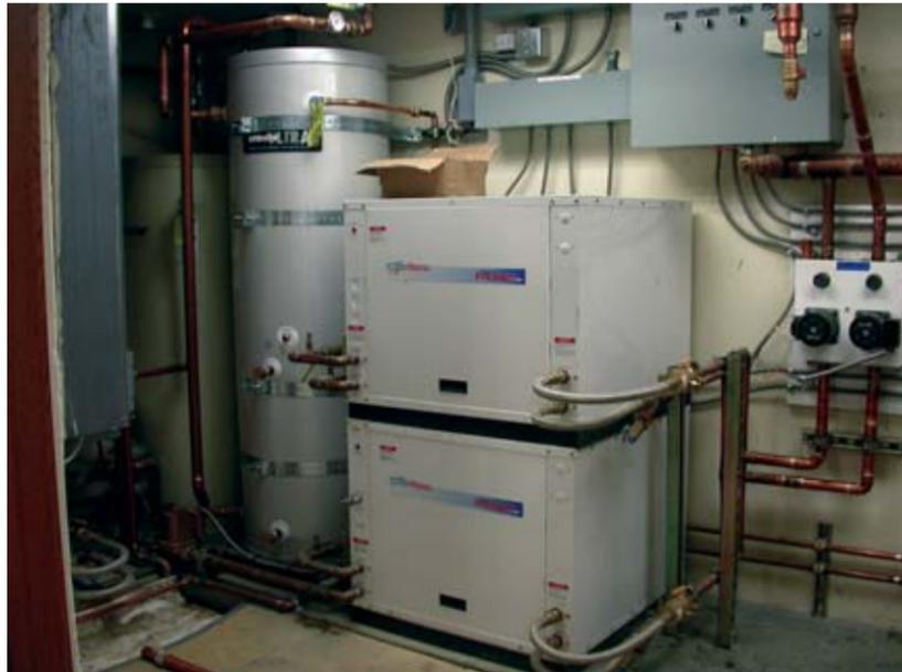
Shown is a typical water-to-water heat pump installation for a radiant floor system. The hot water heater to the left is used as a buffer tank for the radiant floor system.
