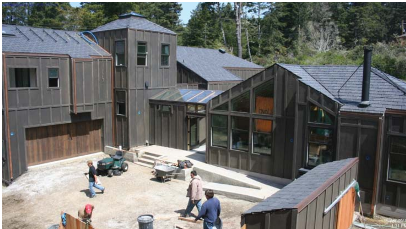
iBeam Time-lapse Pro Construction Camera Perspective 2010-04-15
