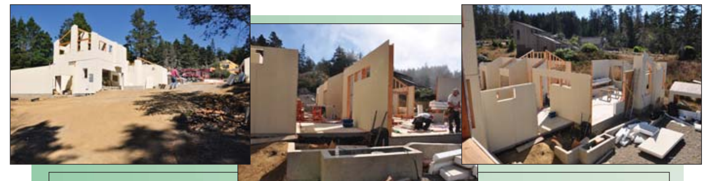
SIP Wall Construction
