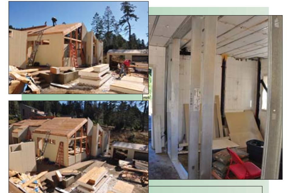
SIP Roof Installation & Deitrich UltraSTEEL® Framing
