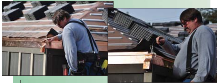
Contractor Roger Stevenson Installing Reeve/CopperCraft Gutters
