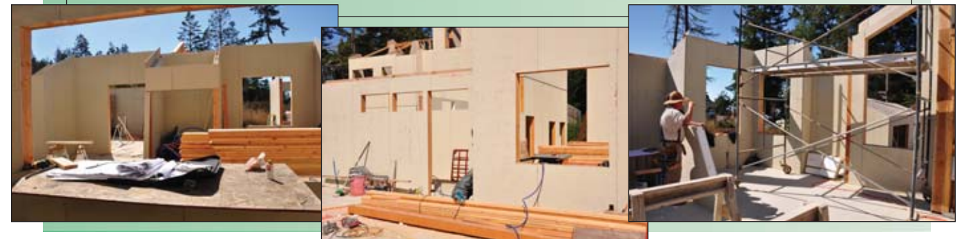
SIP Wall Construction
