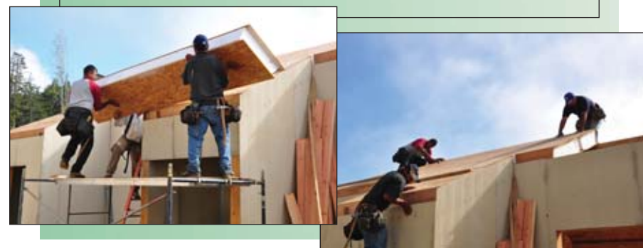
SIP Roof Fabrication & Installation
