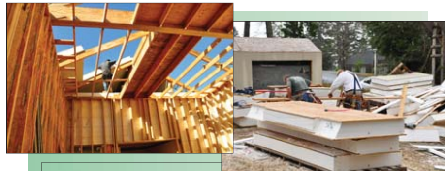
SIP Roof Fabrication & Installation
