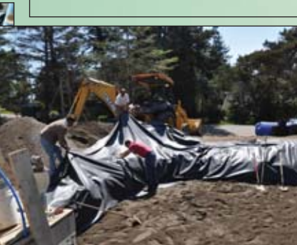
Conservation Technology Mechanical Filter And Electronic Submersible Pump, Heavy Duty .6-Mill-Thick Non-Woven Geotextile Protection Fabric Liner, And Firestone Specialty Products .45-Mill-Thick EPDM PondGuard™ Geomembrane
