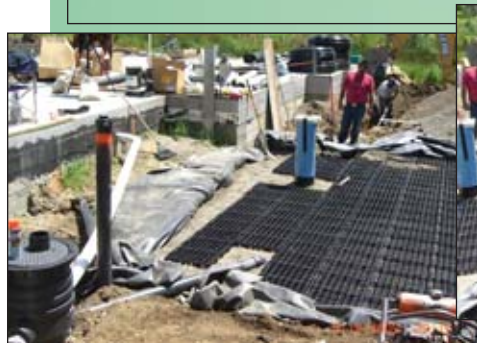
Aqua Nueva's Terry McMains And Crew Installing Stormwater Solutions' EcoRain Stormwater Tank Modules' Underground 2,400-Gallon Water Cistern With Heavy Duty .6-Mill-Thick Non-Woven Geotextile Protection Fabric Liner And Firestone Specialty Products .45-Mill-Thick EPDM PondGuard™ Geomembrane
