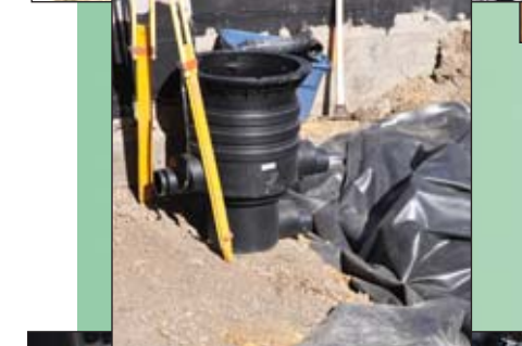
Conservation Technology Mechanical Filter And Electronic Submersible Pump, Heavy Duty .6-Mill-Thick Non-Woven Geotextile Protection Fabric Liner, And Firestone Specialty Products .45-Mill-Thick EPDM PondGuard™ Geomembrane
