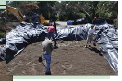
Conservation Technology Mechanical Filter And Electronic Submersible Pump, Heavy Duty .6-Mill-Thick Non-Woven Geotextile Protection Fabric Liner, And Firestone Specialty Products .45-Mill-Thick EPDM PondGuard™ Geomembrane
