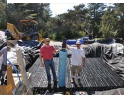
Conservation Technology Mechanical Filter And Electronic Submersible Pump, Heavy Duty .6-Mill-Thick Non-Woven Geotextile Protection Fabric Liner, And Firestone Specialty Products .45-Mill-Thick EPDM PondGuard™ Geomembrane
