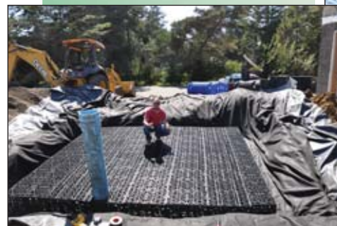
Aqua Nueva's Terry McMains And Crew Installing Stormwater Solutions' EcoRain Stormwater Tank Modules' Underground 2,400-Gallon Water Cistern With Heavy Duty .6-Mill-Thick Non-Woven Geotextile Protection Fabric Liner And Firestone Specialty Products .45-Mill-Thick EPDM PondGuard™ Geomembrane
