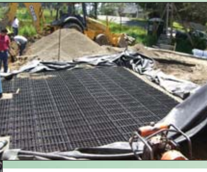
Aqua Nueva's Terry McMains And Crew Installing Stormwater Solutions' EcoRain Stormwater Tank Modules' Underground 2,400-Gallon Water Cistern With Heavy Duty .6-Mill-Thick Non-Woven Geotextile Protection Fabric Liner And Firestone Specialty Products .45-Mill-Thick EPDM PondGuard™ Geomembrane
