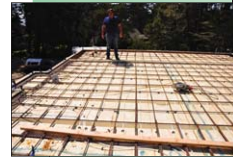
Contractor Roger Stevenson, Brother Dean, And Crew Working With Uponor® AQUAPEX® Embedded Over Amvic® AmDeck® ICF Floor
