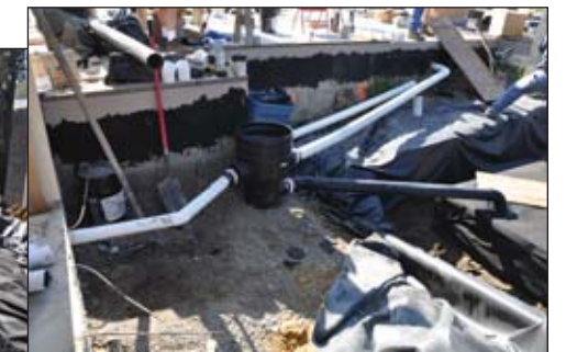
Conservation Technology Mechanical Filter And Electronic Submersible Pump, Heavy Duty .6-Mill-Thick Non-Woven Geotextile Protection Fabric Liner, And Firestone Specialty Products .45-Mill-Thick EPDM PondGuard™ Geomembrane
