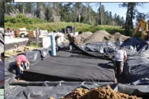
Aqua Nueva's Terry McMains And Crew Installing Stormwater Solutions' EcoRain Stormwater Tank Modules' Underground 2,400-Gallon Water Cistern With Heavy Duty .6-Mill-Thick Non-Woven Geotextile Protection Fabric Liner And Firestone Specialty Products .45-Mill-Thick EPDM PondGuard™ Geomembrane
