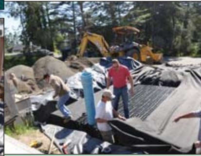
Aqua Nueva's Terry McMains And Crew Installing Stormwater Solutions' EcoRain Stormwater Tank Modules' Underground 2,400-Gallon Water Cistern With Heavy Duty .6-Mill-Thick Non-Woven Geotextile Protection Fabric Liner And Firestone Specialty Products .45-Mill-Thick EPDM PondGuard™ Geomembrane
