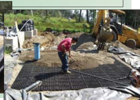
Aqua Nueva's Terry McMains And Crew Installing Stormwater Solutions' EcoRain Stormwater Tank Modules' Underground 2,400-Gallon Water Cistern With Heavy Duty .6-Mill-Thick Non-Woven Geotextile Protection Fabric Liner And Firestone Specialty Products .45-Mill-Thick EPDM PondGuard™ Geomembrane
