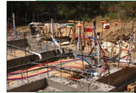
Laying out Uponor AQUAPEX plumbing infrastructure under slab
