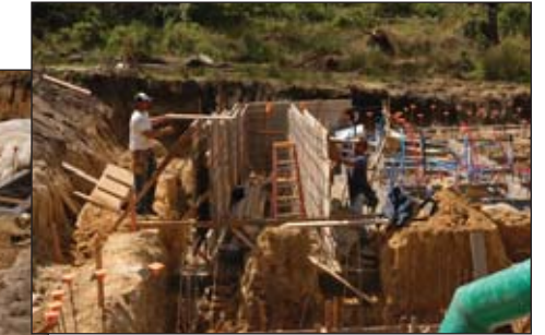
Forming wine cellar and retaining wall/planter
