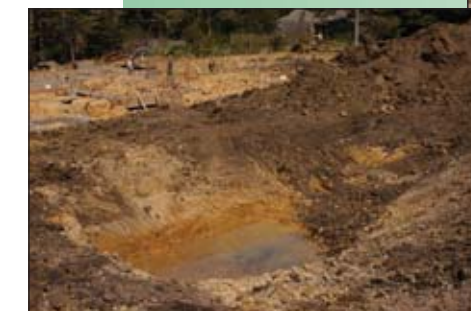
Affluent transfer pipeline crossing road; initial stage of pond excavation
