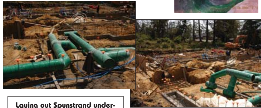
Laying out Spunstrand underground air-conditioning duct
