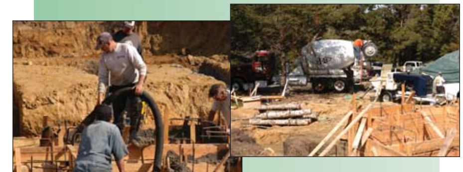
Pouring the concrete in a portion of the standard foundation footings
