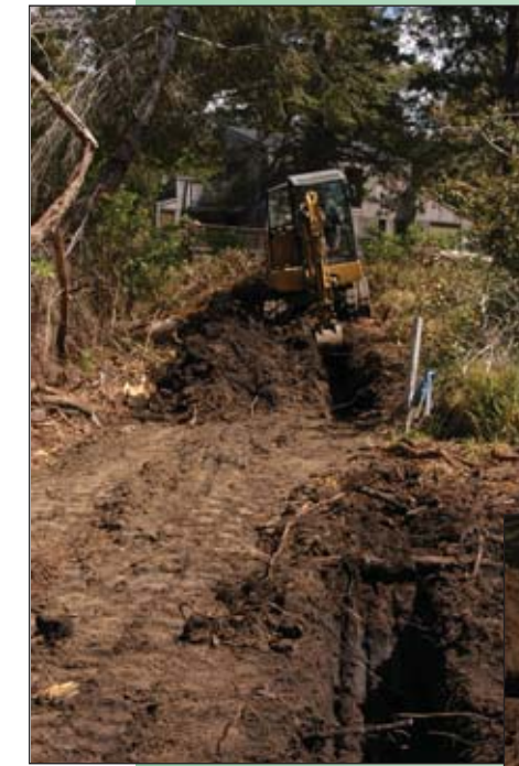
Excavation of septic tank affluent transfer pipeline route
