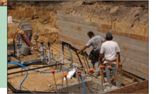
Laying out Uponor AQUAPEX plumbing infrastructure under slab
